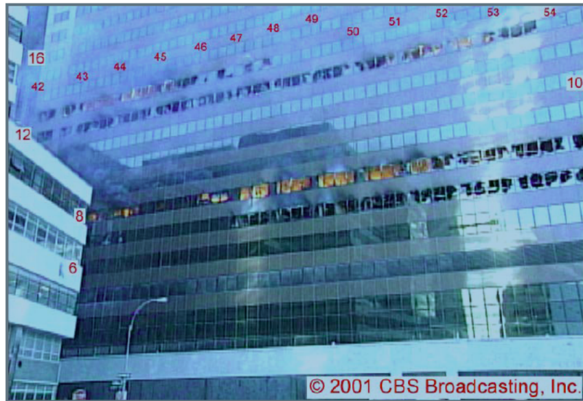
Figure 5-136. Frame taken from a video shot from near the corner of Greenwich Street and Park Place showing the north face of WTC 7 between 3:49 p.m. and 3:54 p.m. The building on the left is 30 West Broadway. The intensities have been adjusted, and column and floor numbers have been added.
